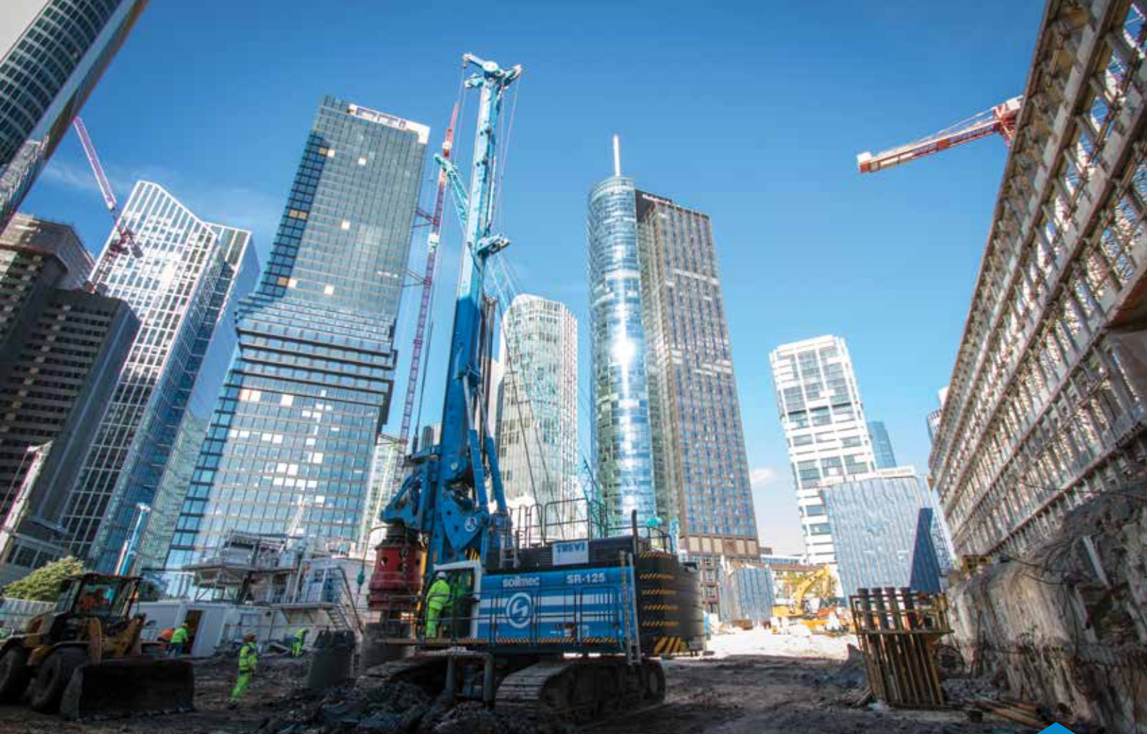
FIGURE 6: EXECUTION OF PILES WITH SOILMEC SR-125
