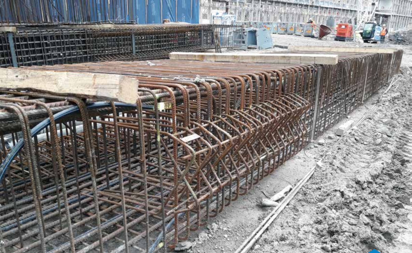
FIGURE 7: OVERLAP REINFORCEMENT
